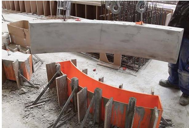
For a building renovation, NOWLAB helped construction company Geiger to reduce costs and time in creating large concrete casting molds.
